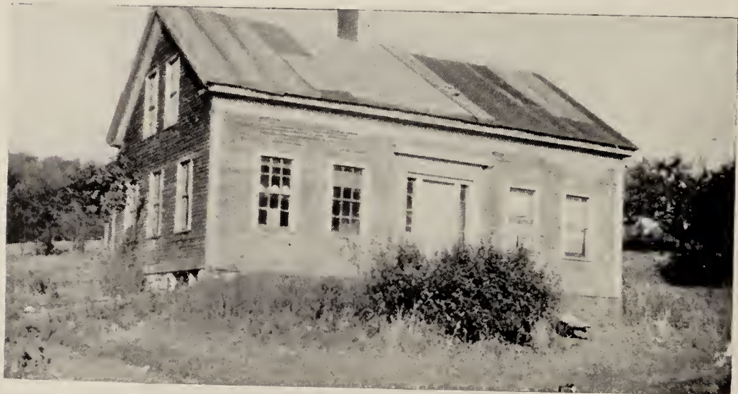
THE GAMALIEL WALDO HOUSE Middletown Springs, Vermont
