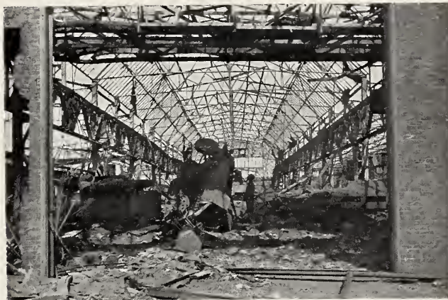
Allied bombing wrecked this factory in Bad Oeynhausen.
