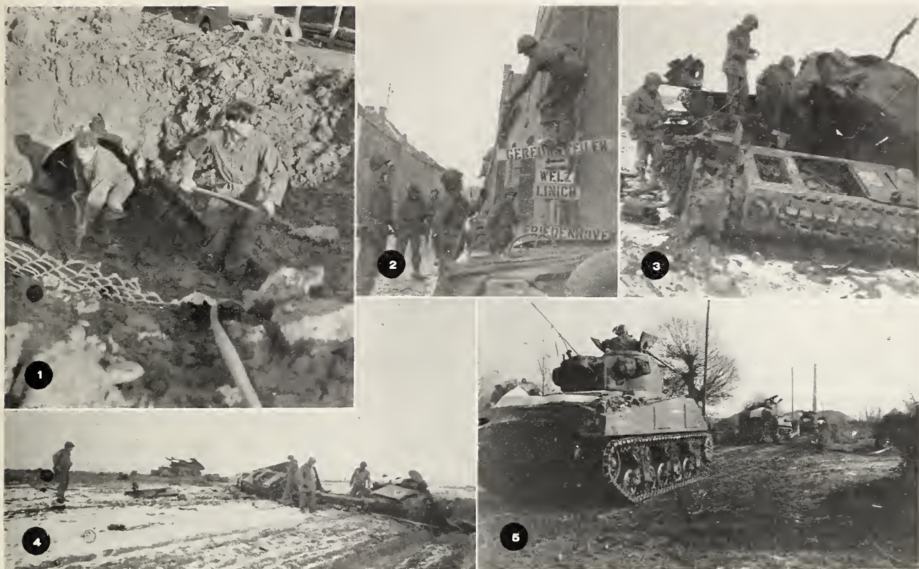
1—Road repair near Ederen. 2—Ederen corner. 3—327th Engineers prepare to demolish a German tank. 4—After the Apweiler battle. 5—2d Armored moves through Beggendorf.
