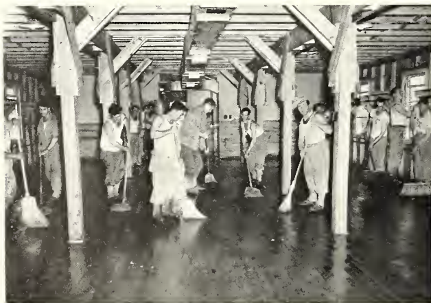
Cleaning barracks inside
