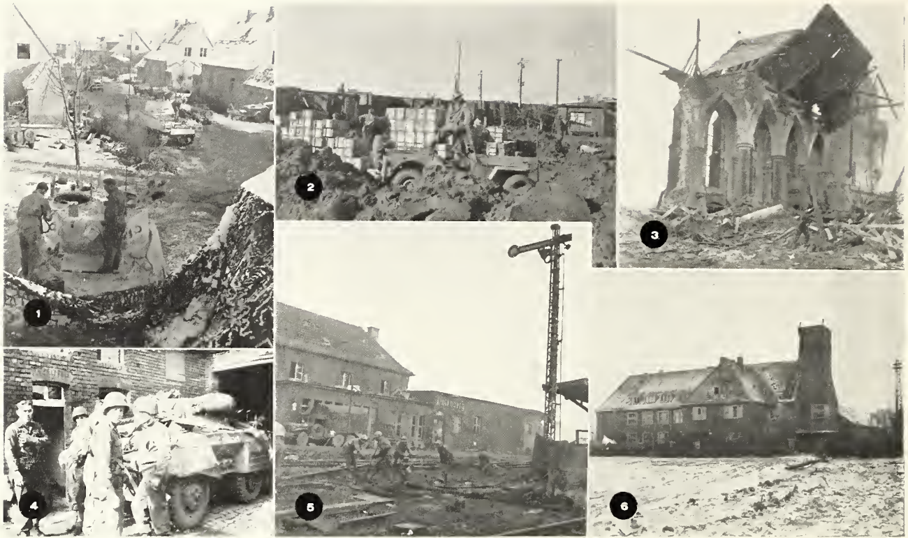
1—Armor is painted white and serviced before moving up. 2—Palenberg railhead. 3—Gereonsweiler church. 4—Recon Troop headquarters. 5—Palenberg, winter home of 102d service units and rear echelon. 6—Division command post at Ubach.
