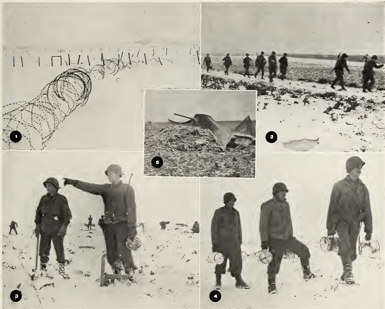
1—The front line. 2, 3, and 4—327th Engineer Combat Battalion laying mines and booby traps. 5—Dummy tank.
