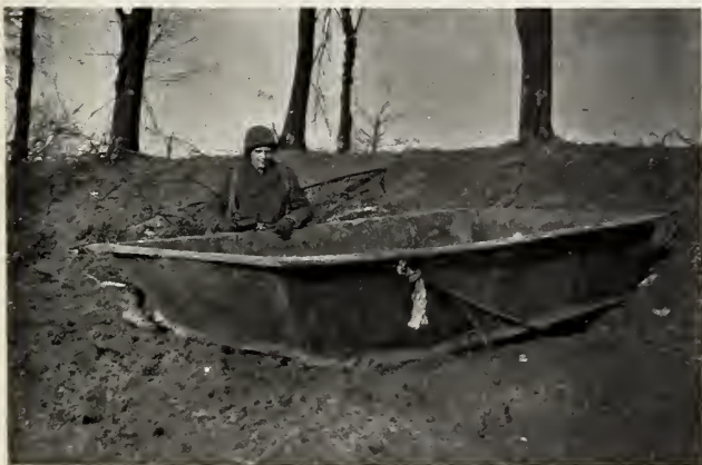
Buck Rogers and the first boat across the river are sheltered by the dike in the background.
