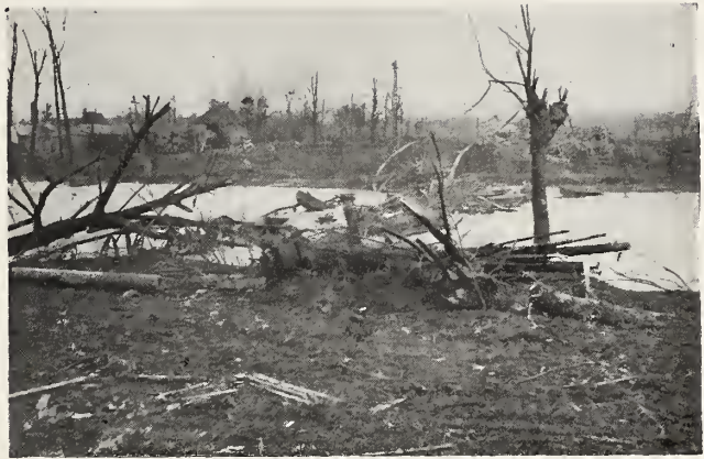
Debris after the crossing.
