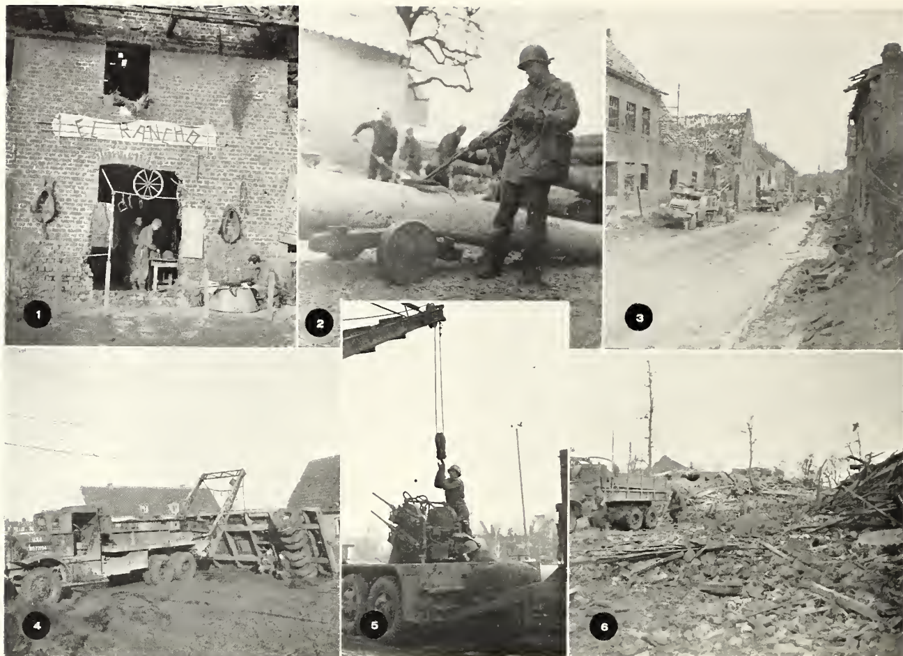
1—406th Infantry armorer-artificer sets up in Gereonsweiler. 2—Local bridging materials were assembled. Hunting shrapnel fragments with a mine detector before sawing the logs. 3—Ederen was a boom town. 4—Cobblestone roads disappeared under heavy traffic. 5—Equipment was overhauled. 6—Six buildings occupied this site before a bangalore torpedo dump exploded.
