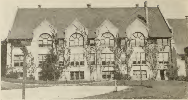
SMITH HALL, THE RECITATION BUILDING
