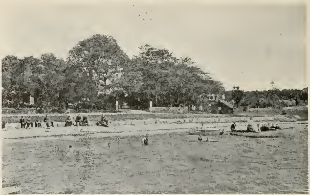
BATHING BEACH AND BOATS, MAIN ENTRANCE IN BACKGROUND
