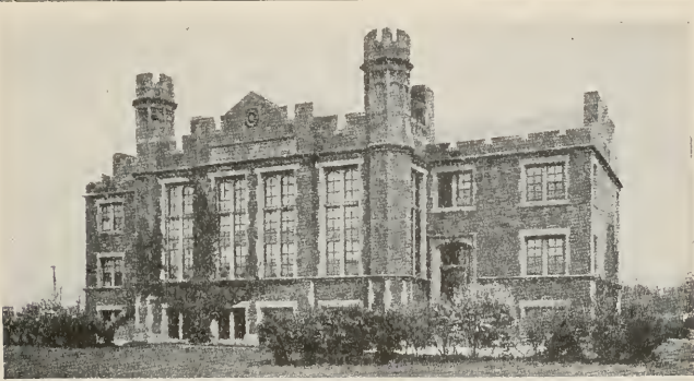
MAIN ACADEMY BUILDING
