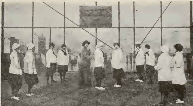
THE ROOF GYMNASIUM
