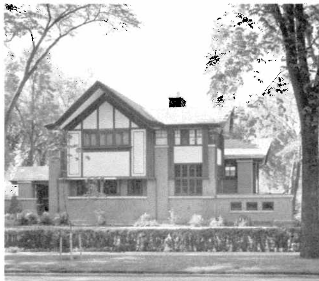
The Emery house (1902) in Elmhurst, Illinois was an important design in Griffin's early career. It employs features found in the 104th Place houses including the high pitched gable roofs, the dark-stained wood detailing under the eaves, and the placement of rooms at right angles to the main axis of the structure. (Richard Nickel, photographer. Courtesy of the Richard Nickel Committee)
