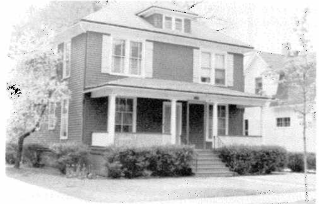
The house at 1703 West 104th Place (above), built in 1910, and the Blount house at 1724 West 104th Place (below), built in 1911, are alike in their size and scale and in their use of balloon-frame construction.
